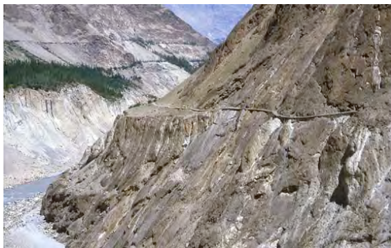
Left: Clinging to the cliff face, some parts of the old Hunza Road are less than two feet wide.
