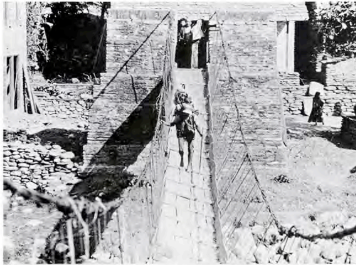
9 Suspension bridges have replaced dugout canoes on most river crossings. Although undoubtedly more secure, they can still provide a challenge to timid travellers – and an entertaining spectacle for the locals.
